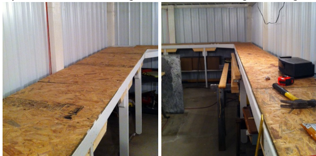
Benchwork mounted on the south & north side walls; respectively
